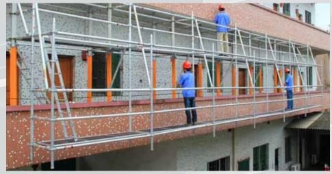
▲ The prop system utilized with Leader GN50 Modular Aluminium Scaffolding System to form suspended facade scaffolding system perfectly for wall construction and refurbishing purposes.
